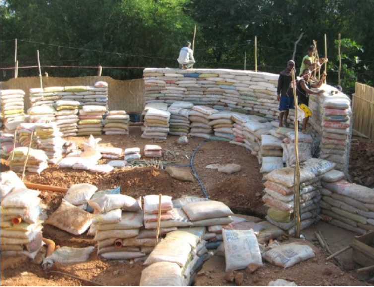
Illustration 8: Sandbag Construction
