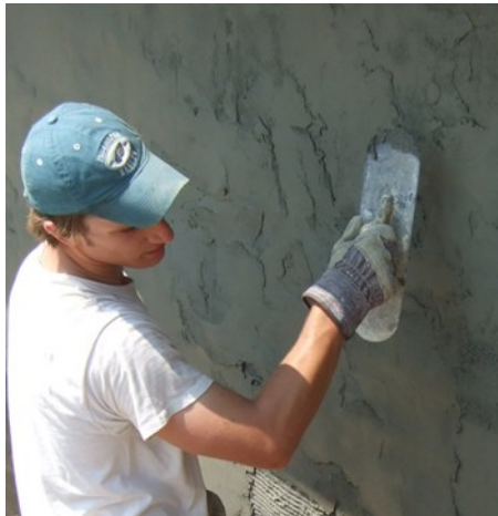
Illustration 13: Applying Stucco
