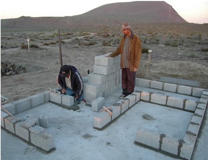
Illustration 10: Cinder Block Construction
