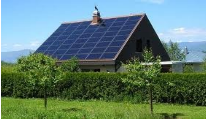
Illustration 16: Solar Roof Panels
