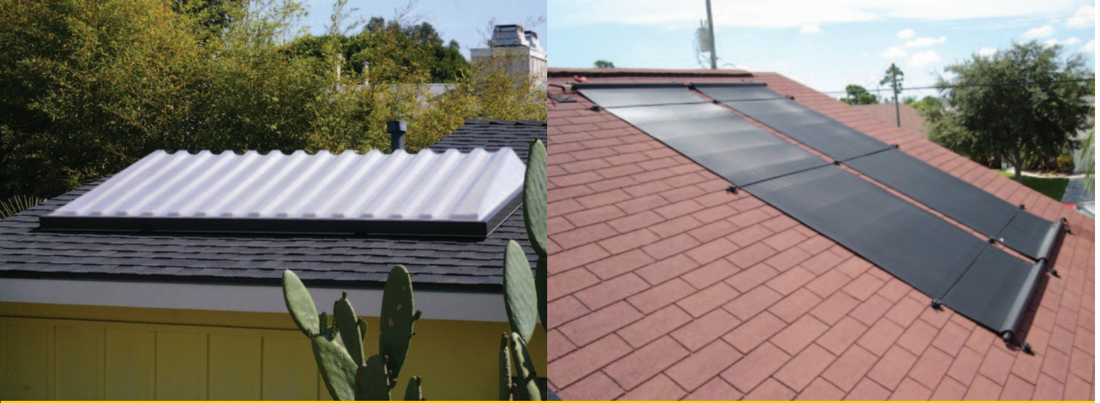
Two U.S.-manufactured low-cost plastic packaged systems are now available, including the SunCache system (above left) and the FAFCO system (above right). The manufacturers use plastic materials that reduce production and installation costs. Photos from Harpiris Energy and FAFCO
