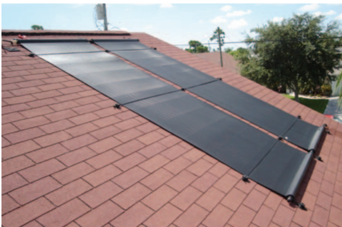
Fig. 7. FAFCO solar water heating systems can be rolled-out onto the roof during installation. The systems are freeze tolerant, do not overheat, and can be used virtually anywhere in the United States. With unglazed collectors such as these, winter performance will be low or non-existent in cold and windy climates. A two-panel drainback system (FAFCO Series 200, shown on the left), providing 48 ft 2 of collector or, (right) A four-panel drainback system, providing 96 ft 2 of collector area. Both systems have a very low profile compared to conventional collectors. Photos from FAFCO
