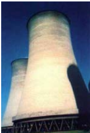
Zambia Cooling Towers Industrial Water Cooling Ltd
