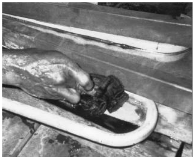
5: Then cool down the solder joint of pipe and sheet with damp cloths and next to remove the superfluous soldering flux.
