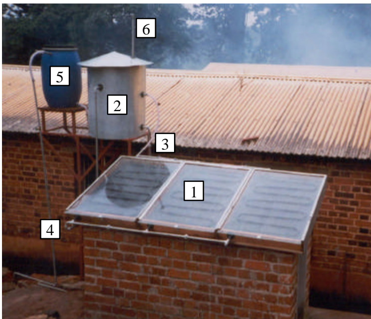
A complete solar hot water system, installed at Hospital Peramiho.
